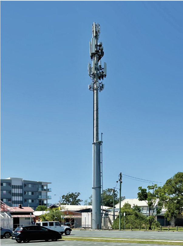
Fig. 2. This 5G base station in Australia receives signals from users' cell phones and passes them on to the network core so they can be routed to their destinations. Some 5G frequencies require large numbers of base stations in a small area because of interference from buildings and other objects in the environment. Credit: Kgbo/Wikimedia Commons (CC BY-SA 4.0).
