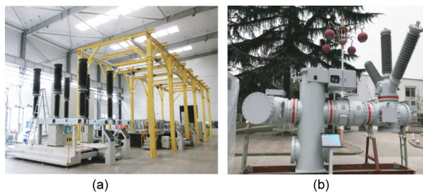
Fig. 1. Eco-friendly 126 kV VCBs. (a) Baosheng Group (China), a product line of live-tank single-break 126 kV, 3150 A, 40 kA VCB with 0.2 MPa N 2 as the external insulation medium of the VIs; (b) Pinggao Group Corporation (China), 126 kV, 2500 A, 40 kA vacuum GIS with 0.5 MPa CO 2 as the external insulation medium of the VIs [26].
