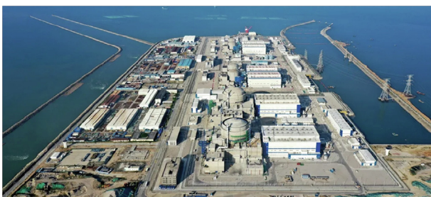
Fig. 1. Aerial view of the first unit of the HPR1000 Demonstration Project in the world: Unit 5 of Fuqing Nuclear Power Plant.
