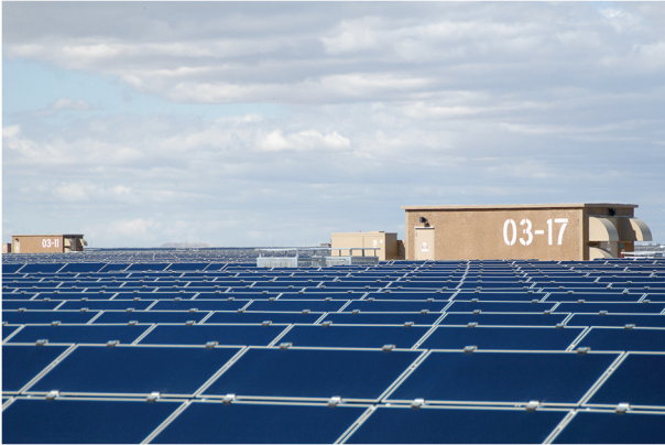
Fig. 1. The cost of generating electricity with renewable sources, such as the solar energy captured by the immense Topaz Solar Farm in San Luis Obispo County, CA, USA, has fallen below the cost of using natural gas. The facility covers 25.6 km 2 and generates 550 MW of energy with nine million thin-film cadmium telluride panels. Credit: Sarah Swenty/USFWS (CC BY 2.0).
